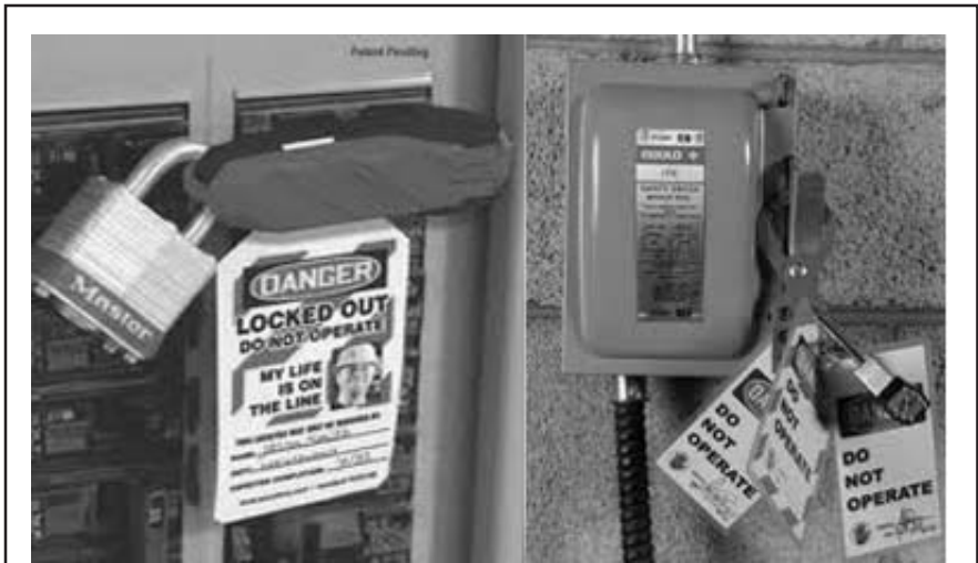
Figure 3: Lockout devices are available in various shapes and sizes that allow for the lockout of standard control devices.
